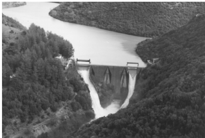
Figure 5: View of Ladon Dam from downstream, showing both spillways in use for the first time since the beginning of the operation of the hydroelectric station in 1955. Photo taken just after the flood period of February 2003.
