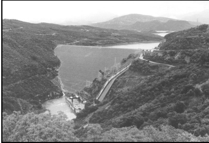
Figure 1: View of the Kremasta Dam from downstream. The spillway and the hydroplant can be seen on the right.
