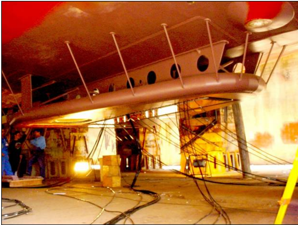
Fig. 3.18 "Gondola installation"
