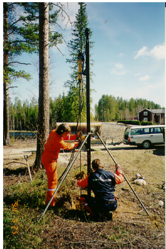
Fig. 4. An underground benchmark is set out.
