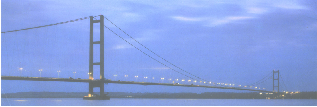
Fig. 1, The Humber Suspension Bridge.
