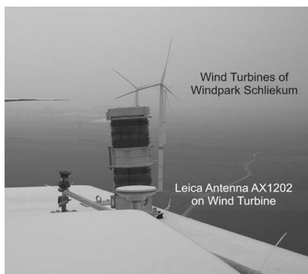
Figure 13: Rover Station on top of the WET
