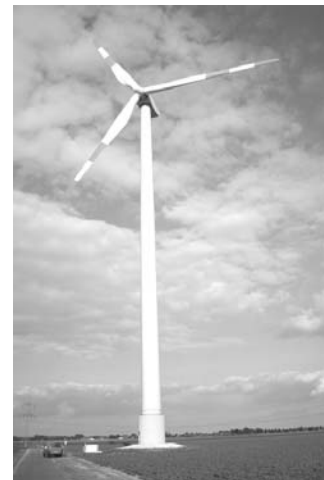
Figure 1: WET in Schliekum, Germany
