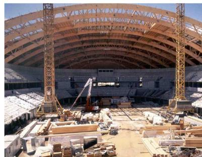
Fig. 4 – The erection of the glulam structure
