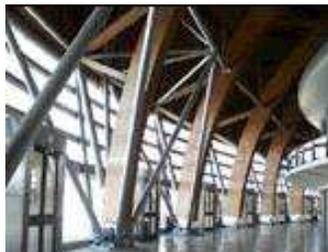
Fig. 3 – The feet of the arches as seen in the deambulatory.
