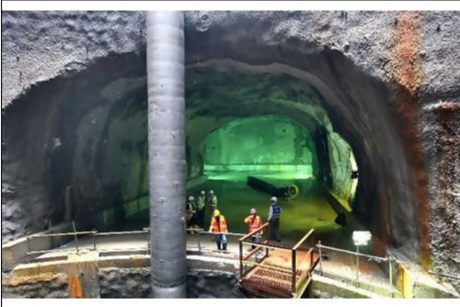
Figure 8. Underground rock cavern development (source: Jurong International)
