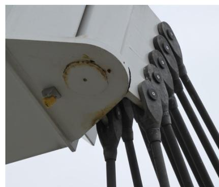
Figure 3. Leica GPR112 prism in the lower part of the rotating head holding the footbridge with the help of cables.
