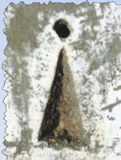
Drill Hole and Wing in Kerb
