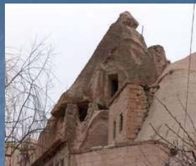
Figure 6: A room curved from rock
