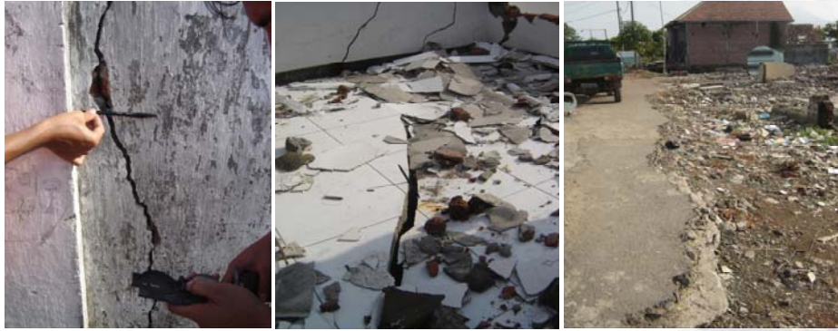
Documentation on cracks on the wall, streets, floor around Renokenongo village
