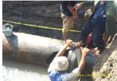
Crashes of Pipe water belong to district water management of Porong Sidoarjo
