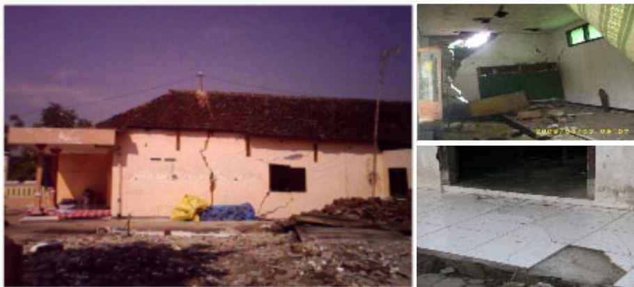
Documentation on cracks on the wall, house, floor around Sengon village
