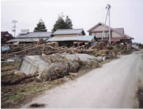
Concrete block walls mowed down by the tsunami
