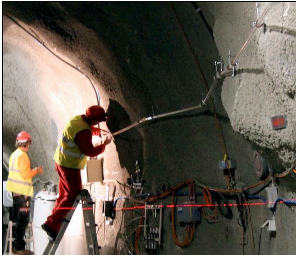
**Fig. 6):** HLS acrylic glass tube installation using a laser beam in the rock laboratory, Gallery 98
