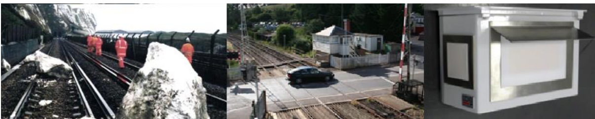
Figure 18 From right to left i) Rock fall obstructing track ii) Sirio system is setup at critical safety zones such as level crossings iii) the Sirio radar for obstacle detection
