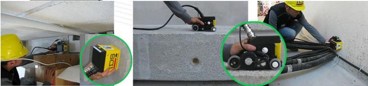
Figure 19 Concrete scanners can be used to assess the condition of concrete structures after major disaster event as a way of risk mitigation
