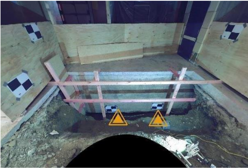
Figure 8 - Pier Cap and Pile Location Survey
