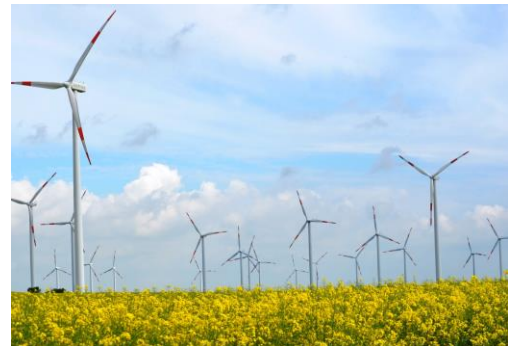
Figure 1. Typical wind turbines
