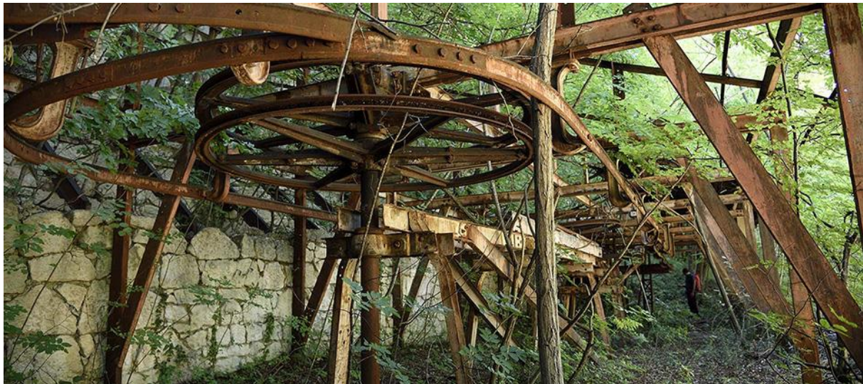
Fig.6 Engine Structure outside the mine
