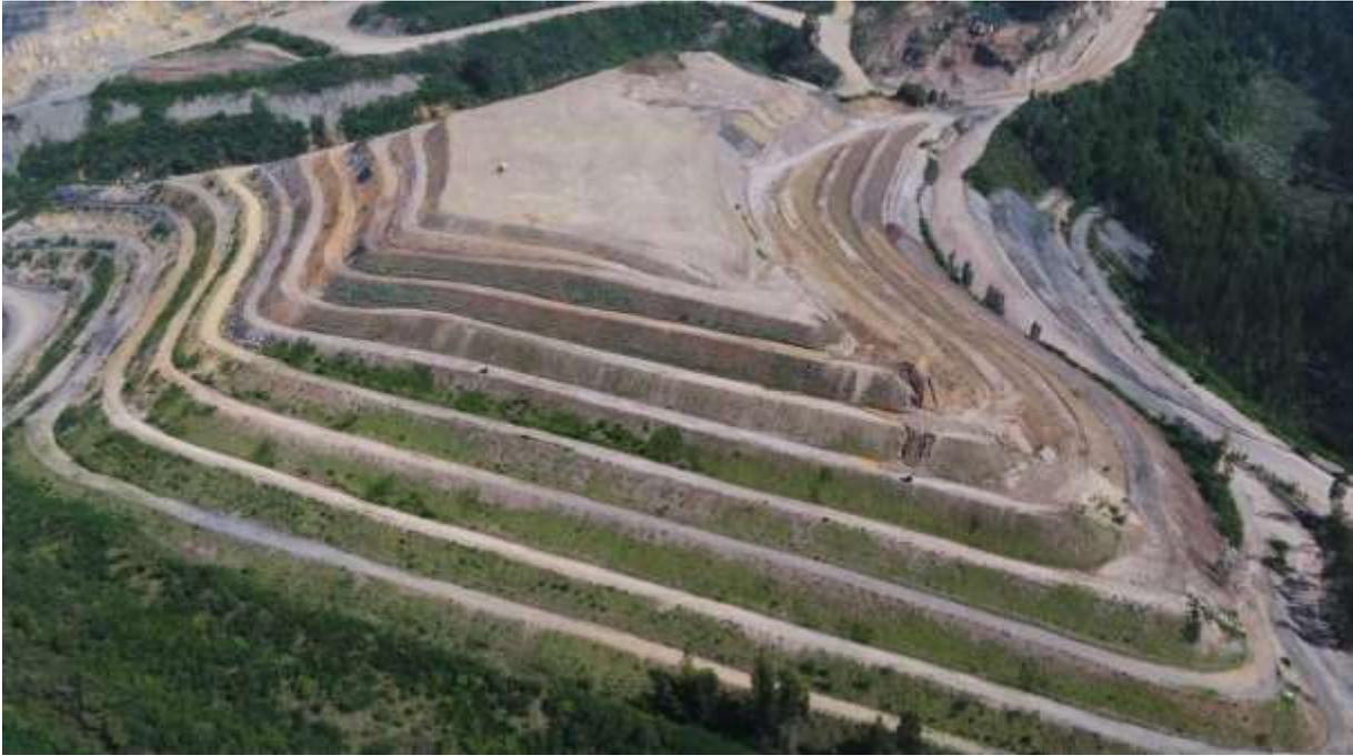
Figure No. 3 Progress of the rehabilitation process Sterile disposal area San Antonio Mine
