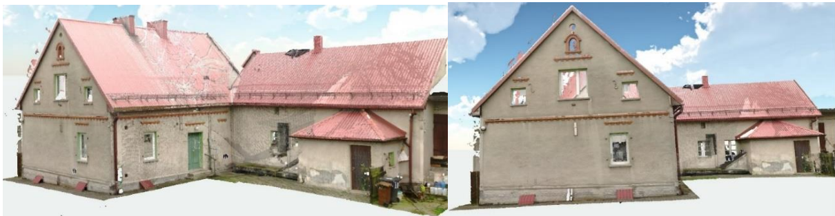
Fig. 7. Three-dimensional model of the object after the processing of point clouds (source: own study)
