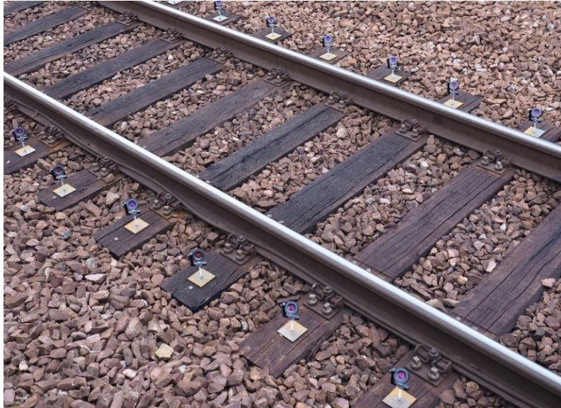
Figure 5 Prisms along the railway track
