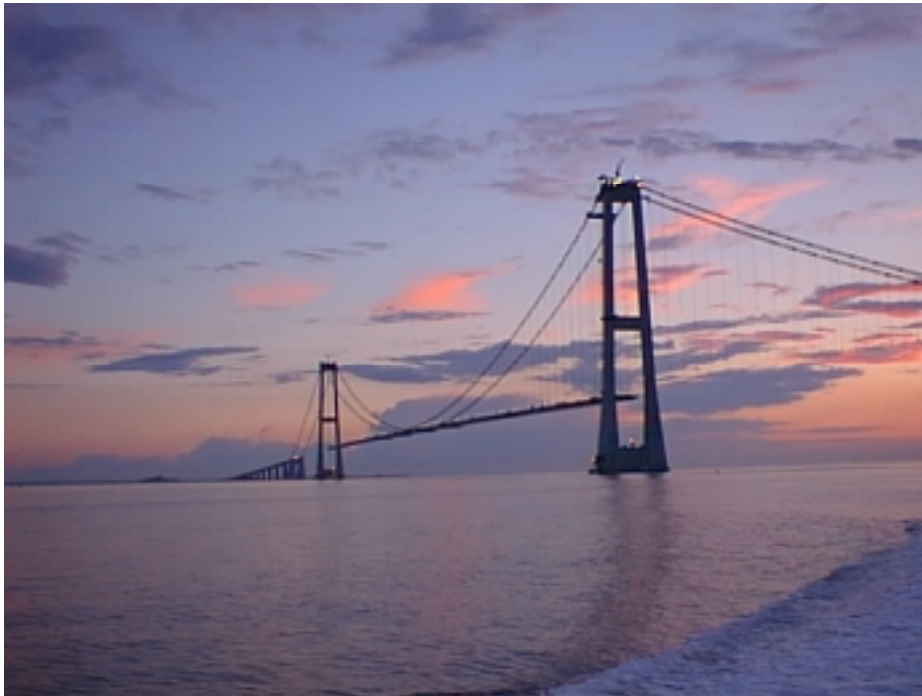
The Bridge for the eastern portion of the Great Belt Fixed Link
