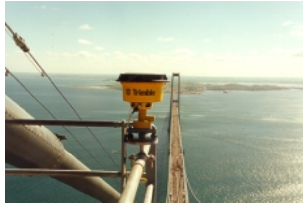
The bridge on a pylon
