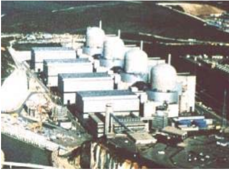
PWR nuclear power plant
