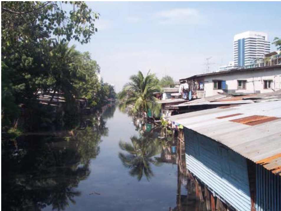
Figure 8: Land rights of people living in slum areas are mostly not recognised or often the situation is considered to be illegal. In any case inclusion in formal land administrations is not possible. Extensions to formal land administrations are urgently needed allowing recordation of all people to land relationships.
