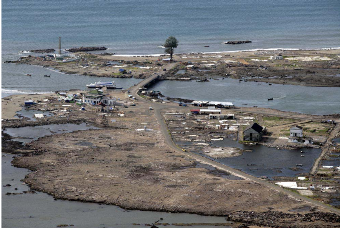
Photo 1. Damaged areas of Aceh
