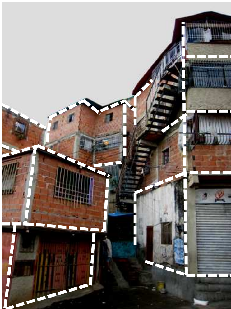
Figure 3 - Improvised housing units in an informal settlement in Caracas, Venezuela Source: © Martim Smolka; rendering by Diego Erba.
