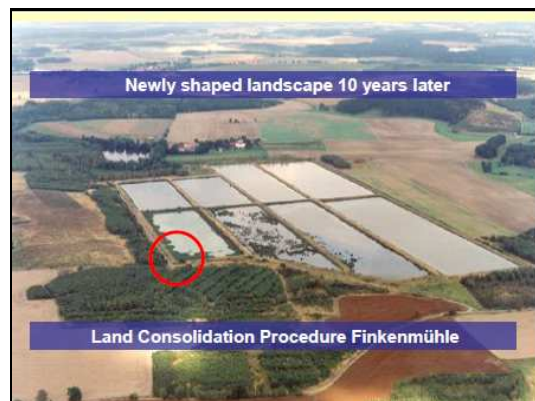
Figure 11. Ecological land consolidation
